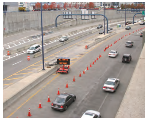
McMahon prepared more than 50 Traffic Management Plans to keep Boston traffic moving during emergency work on the Central Artery/Tunnel and I-90 Connector closure.
