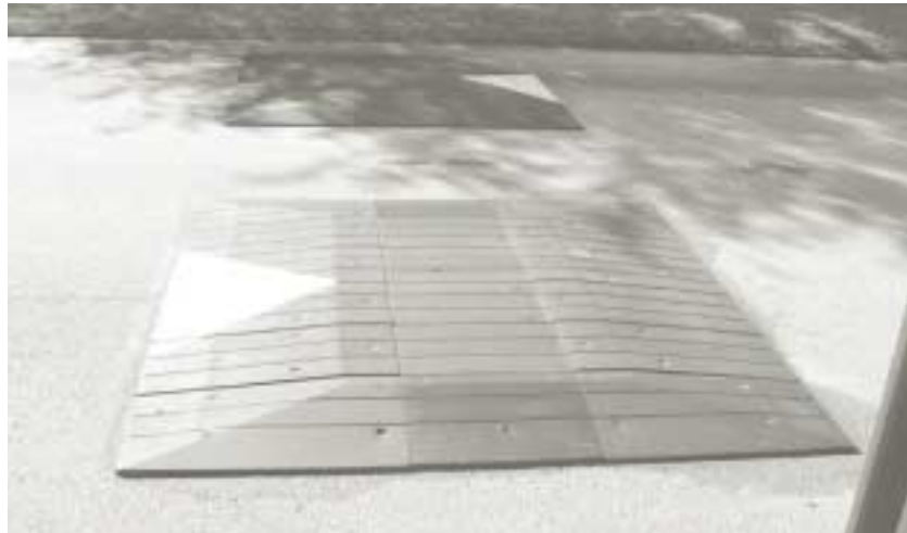
Speed cushions help reduce speeds, but their shape allows emergency vehicles to pass over unaffected.
