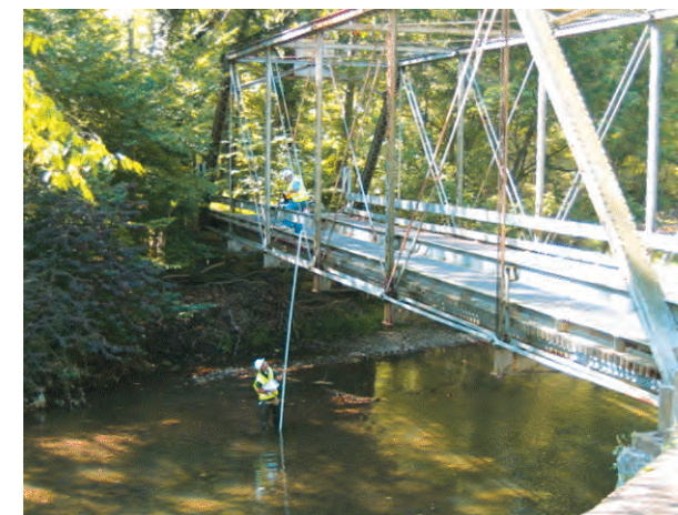
Bridge inspections should be a part of any roadway program.
