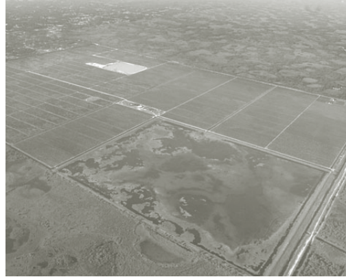
Aerial view of the future site of research institute in Palm Beach County.
